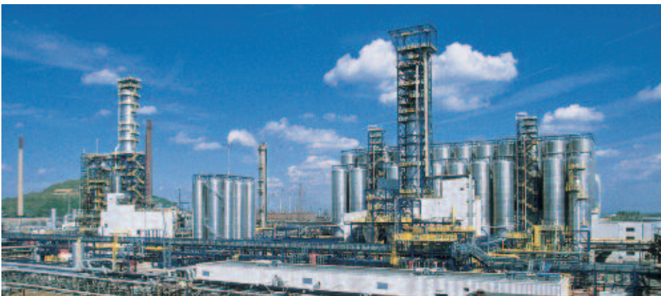
Sabic Polyolefine GmbH production plant at the Gelsenkirchen site
